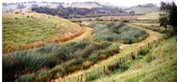
Photo 1: Surface-flow wetlands providing advanced secondary treatment at Kaiwaka after 2-stage waste stabilisation ponds. see also: Additional photos (ca. 90 kB)
