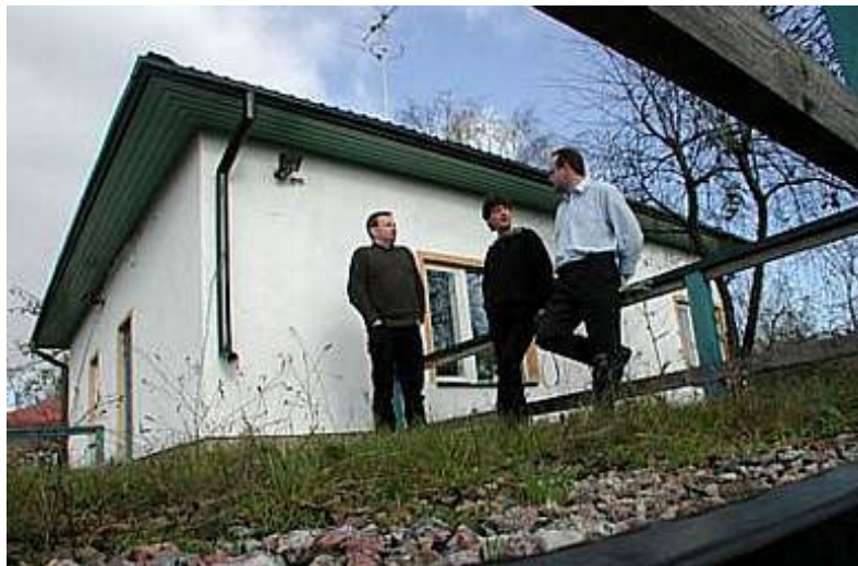
Figure 1: The CEET building in Tartu. On the photo: T.Mauring, J.Heeb and M.Strandbeer (from left to right) Photo: R.Müller
