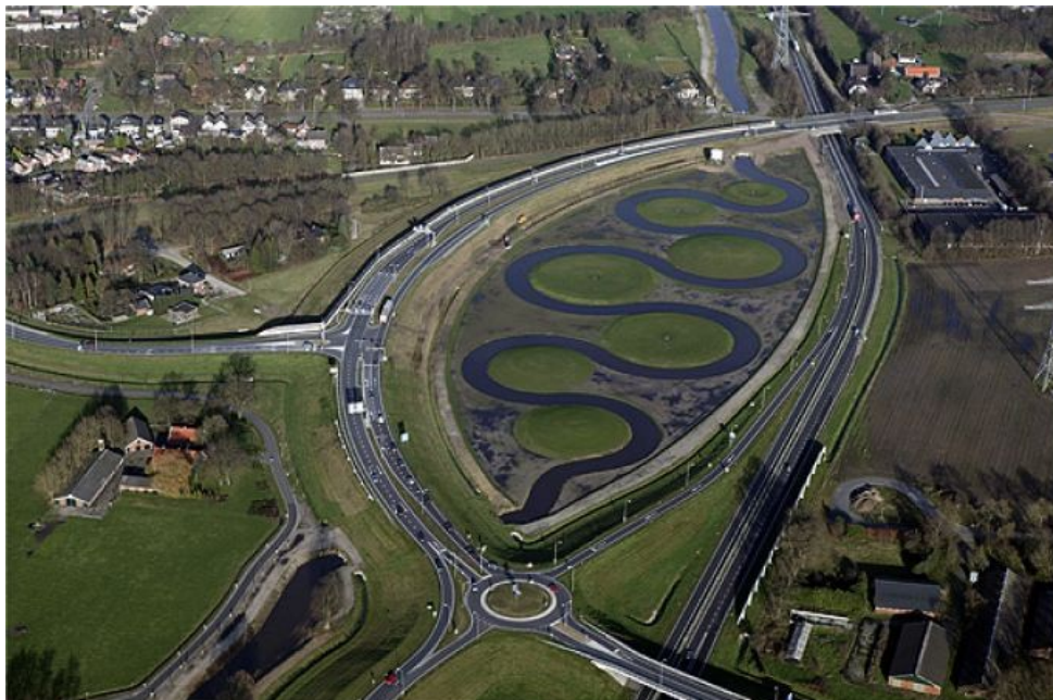
Waterblad: Art and engineering combined for floodwater retention in The Netherlands: Designer: Jeroen van Westen, http://www.jeroenvanwesten.nl/
