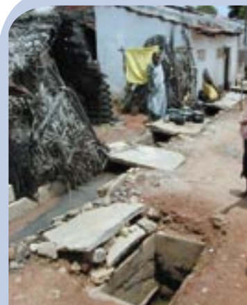
Water well (right) adjacent to an open sewer. Photo: J. Heeb
